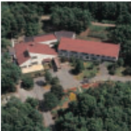
Established in Kobuchizawa in Yamanashi Prefecture in 1981, the KITZ Technical Training Center is the only permanent facility in Japan offering training in valve technology. A large number of our customers use this facility.
